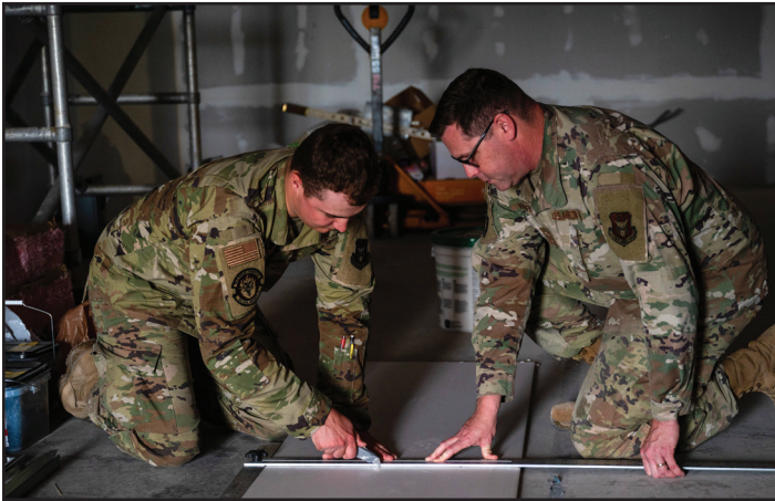
Staff Sgt. Ben Maxfield, 445th Civil Engineer Squadron structural journeyman, right, and Senior Airman Kevin Kruger, 445th CES structural journeyman, cut drywall during a deployment for training at Patrick Space Force Base, Florida, March 5, 2025.
