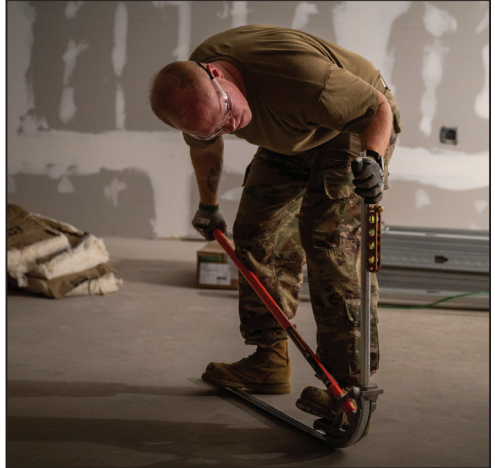
(above) Tech. Sgt. Brandon Gilmore, 445th Civil Engineer Squadron electrical journeyman, bends a pipe while using a level during a deployment for training at Patrick Space Force Base, Florida, March 5, 2025. The deployment for training included Airmen from the 445th CES from Wright-Patterson Air Force Base remodeling a joint warehouse space on PSFB to convert it into office space for the Requirements and Optimization office of the 445th CES.
